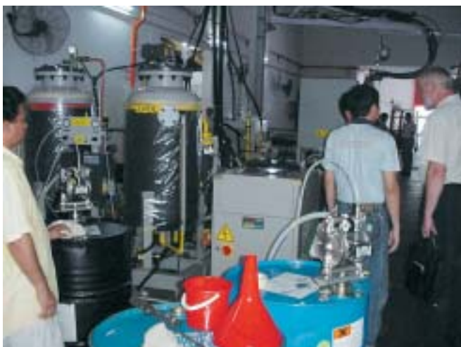
UNDP's Montreal Protocol Unit assists companies converting their operations to use alternative ozone-friendly substances.
